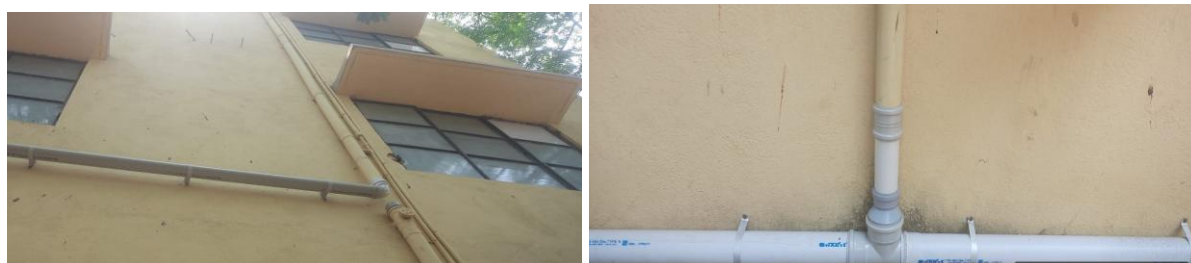
Rainwater collection pipe for Ground water recharging:
